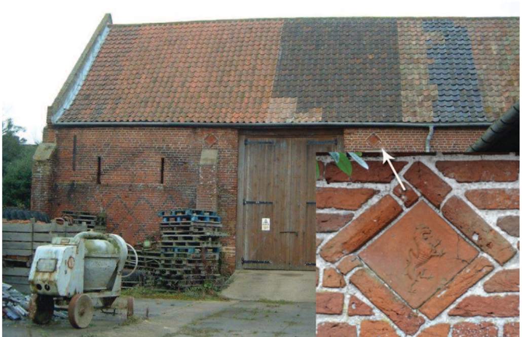
FIG. 55 – The late sixteenth-century barn at Kelsale, with inset of terracotta plaque. The plaques can be seen either side of the doorway above the buttresses ( photos: R. Hoppitt, J. Rainer ).
