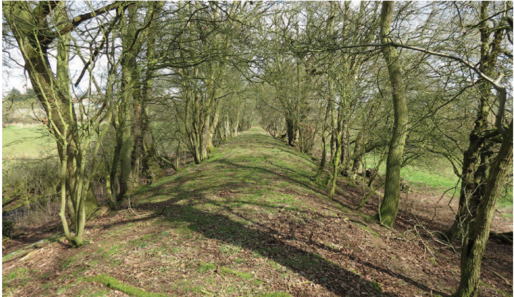
FIG. 58 – The top of the fishpond dam looking north-east ( photo: J. Rainer ).
